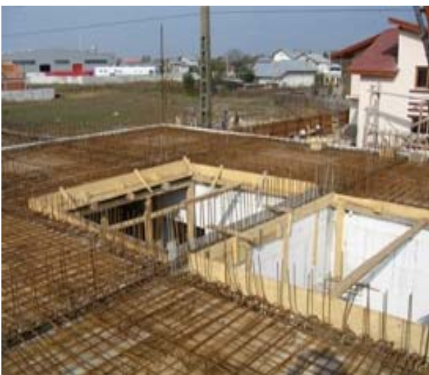
Fig. 3 The reinforce of floors and walls
