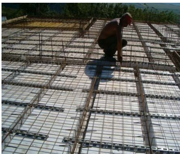
Fig. 5. The reinforce of floors and walls Fig. 6. The reinforce of floors and walls
