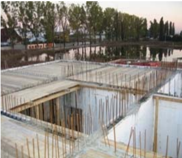
Fig. 1 The cast of walls over foundation
