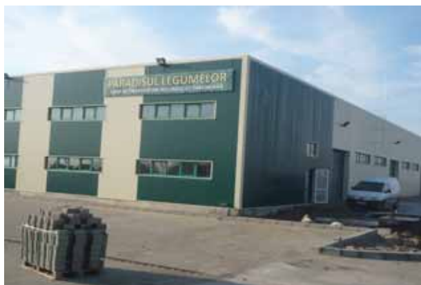
Photo 1. Producer group “SC Paradisul Legumelor Curtici & Macea s.r.l”- space for reception, storage, sorting, packaging, labelling and delivery of vegetable production
