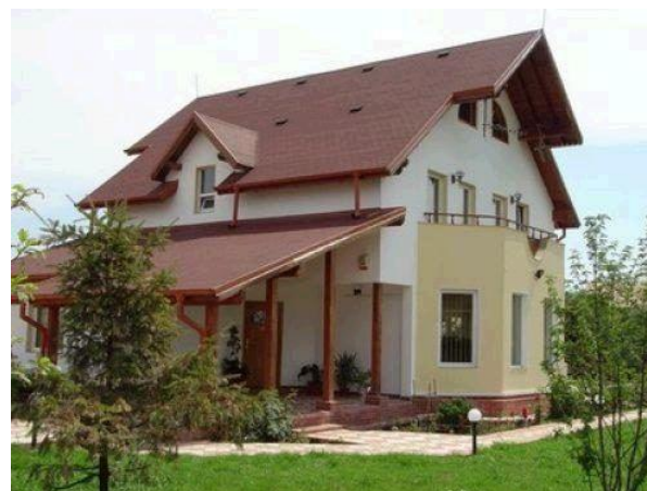
Fig. 4. Ecological house built in Wood Framing System
