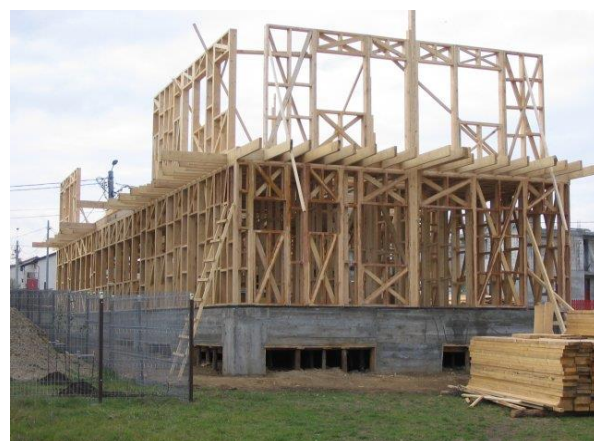
Fig. 2. Foundation and structure of ecological wooden houses
