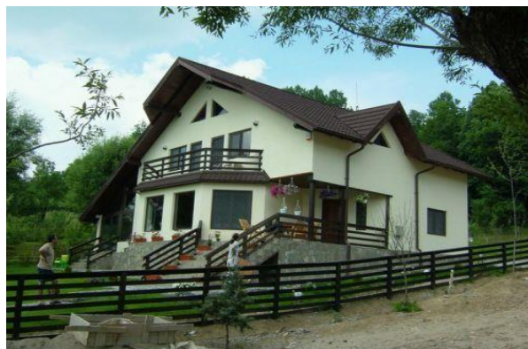
Fig. 3. Ecological house built in Wood Framing System
