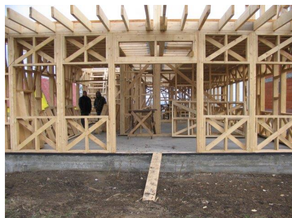
Fig. 1. Structure of ecological house
