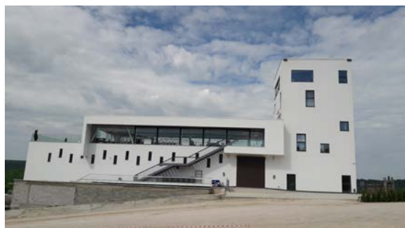
Fig. 6. Poiana Winery. North-east facade (photo A. Trifan, 2019).
