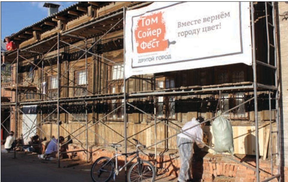
Figure 4. Tom Sawyer Fest. Samara 2018. Restoration in progress Source: https://hinstein.ru/uploads/577417f0537cd.jpg
