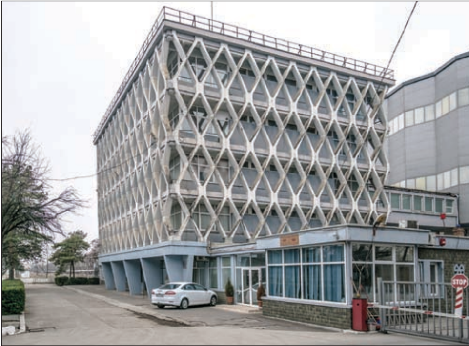
Figure 2. Sugar Factory in Buzau, Romania (BACU Association Photo department, ca. 2015)
