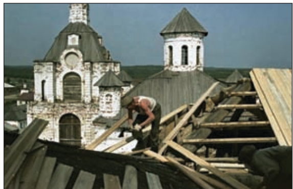
Figure 12. Roof conservation by volunteers. Photo by Vsevolod Tarasevich, 1960
