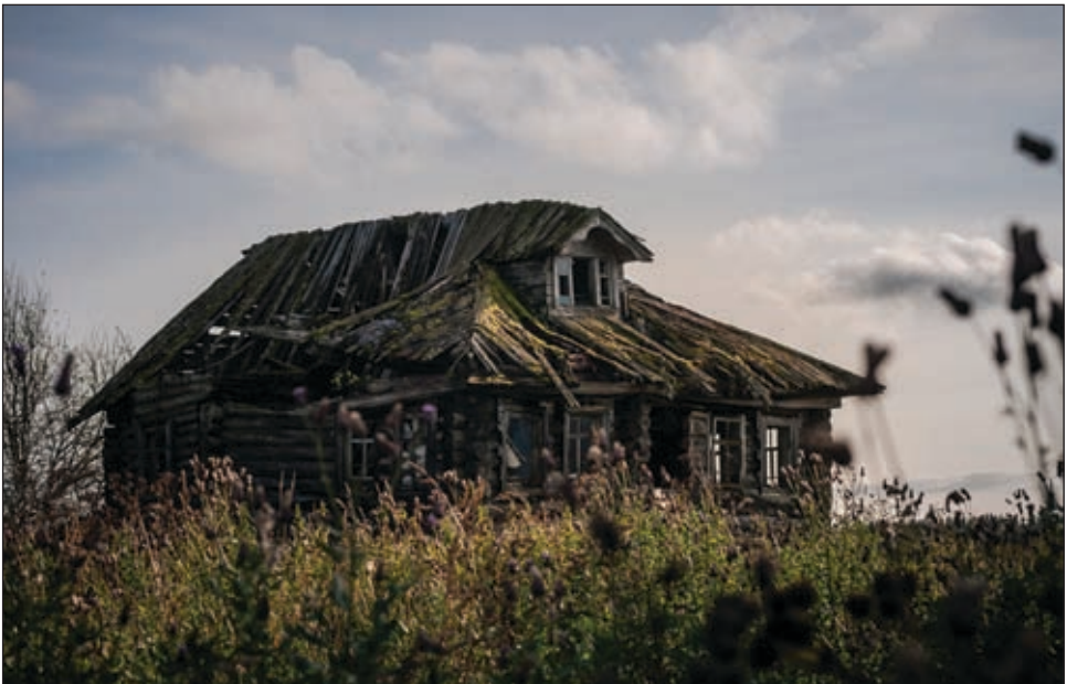
Figure 2. Kuchepalda. House. Photo by Vadim Razumov
