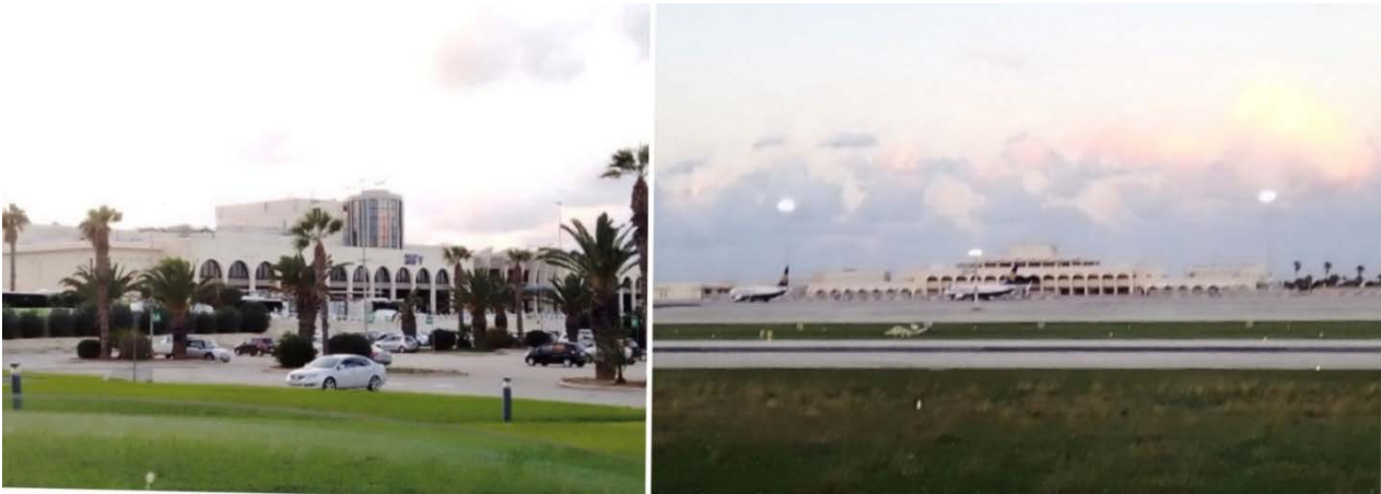
Figure 2. Terminal of MIA (online version is in colour): as at present (left), and as viewed from the side of the runway (right) (© Alessandra Bianco).
