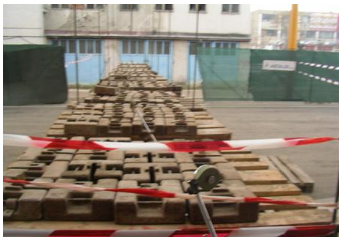
Fig. 4. Equipping set up and service loading.
