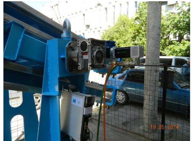
Fig. 8. Elevation motor and drive mounted on the ramp [4]
