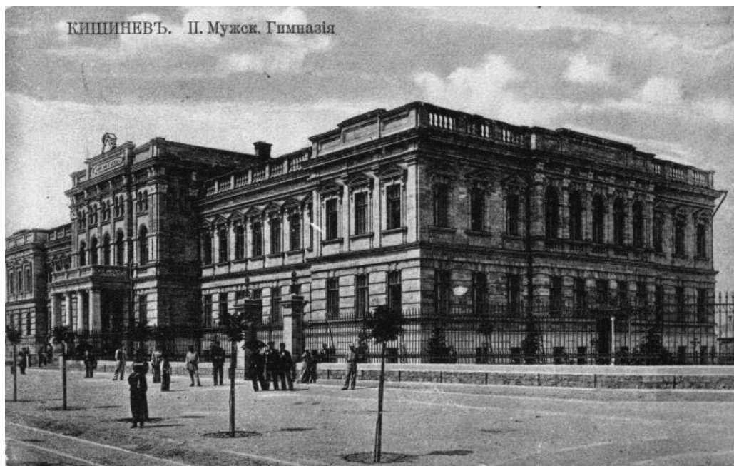
Fig. 1. Chisinau the 2nd male gymnasium's building. The projects for its construction were drawn up by the district architect Demosfen Mazirov. http://oldchisinau.com/
