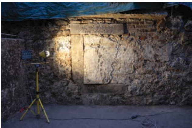
Fig. 10. Latrina in the medieval House Lyverman (City of Cologne)
