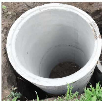
Example of construction of cesspool/ cesspit with reinforced concrete rings
