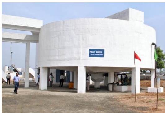
Fig.4 : Elevated Primary Clarifier
